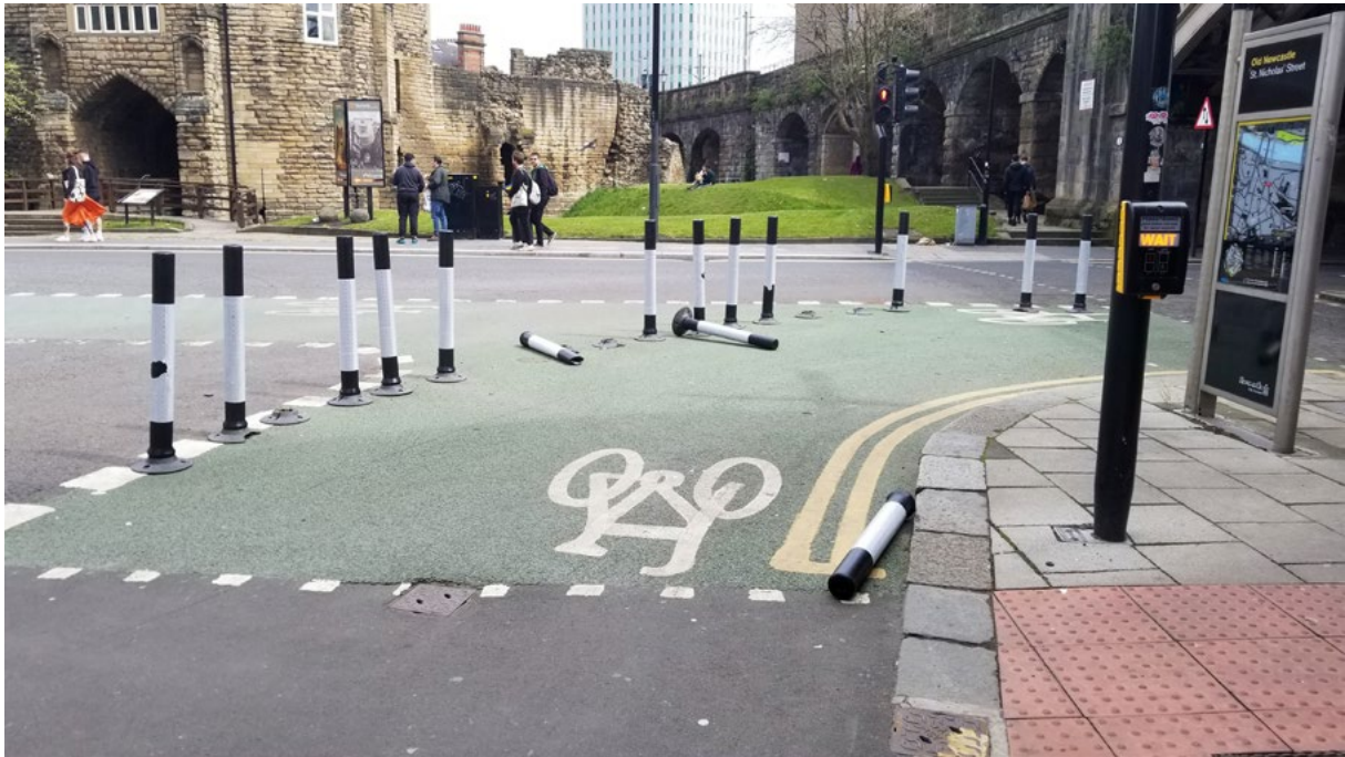
Figure 1: Newly installed bicycle lane in Newcastle, UK. Note the bollards knocked over by vehicles adjusting to the new layout. Source: Author.
